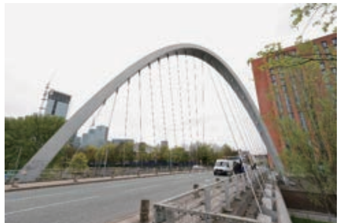
写真－5 Hulme Arch Bridge
