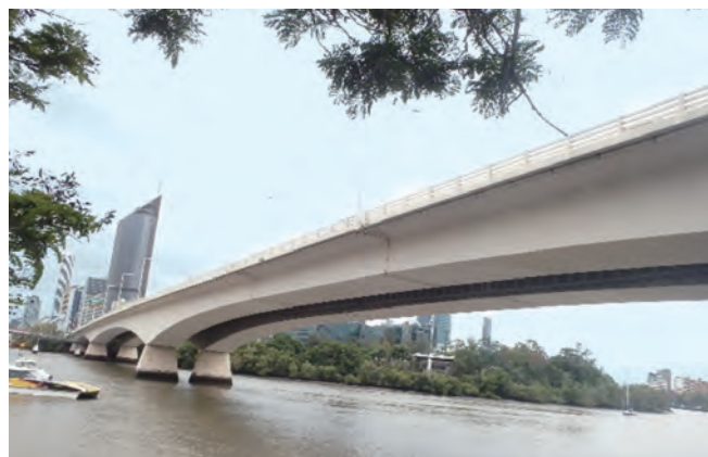
写真-9 Captain Cook 橋
