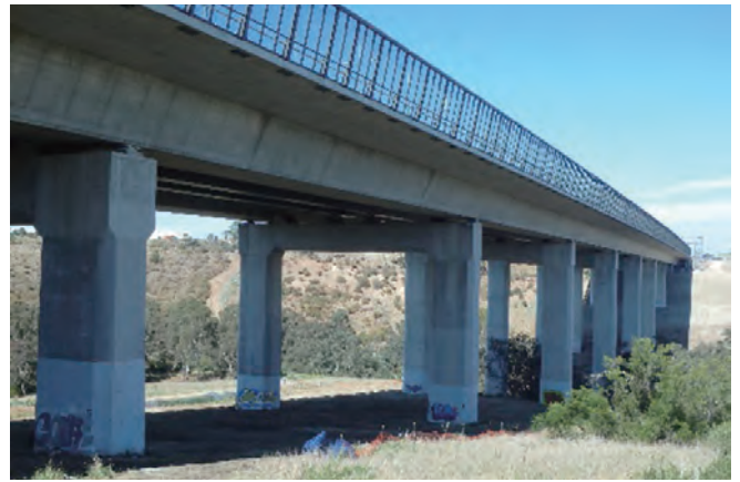
写真-3 Maribyrnong river 橋
