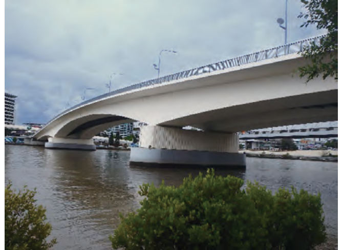
写真-6 Go Between 橋
