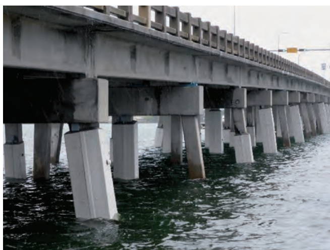
写真-4 Cortez Bridge (RC橋脚柱の電気防食)
