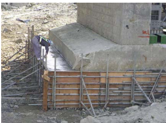
Concrete placing in the scoured part
